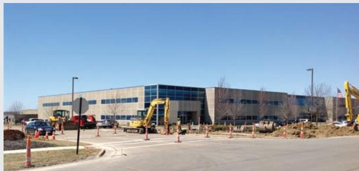
Construction has begun for a traffic signal installation at the intersection of West Tech Road and State Route 741. West Tech Road will be widened to accommodate two left hand turn lanes, northbound, onto State Route 741. South Tech Boulevard will be changed to be a right in/ right out only. The project was awarded to R.B. Jergens Contractors, Inc. Construction is ongoing, and will be completed by the summer.
