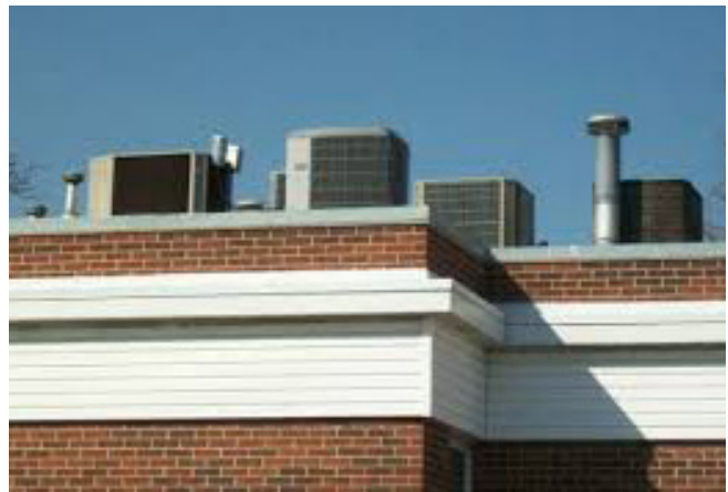
This roofline does not effectively screen rooftop equipment. A parapet wall should be extended up to fully hide the equipment.
