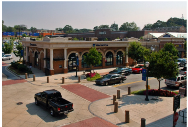
Small turning radius reduces crosswalk distances, while larger turning radius is accommodated with bollards and a flush curb.
