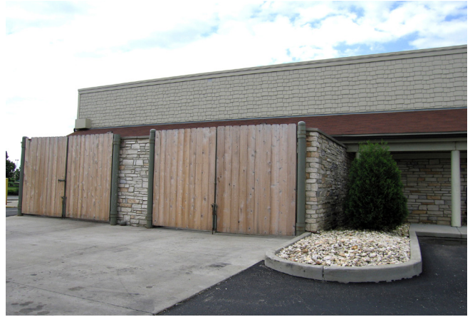
Dumpster are completely screened on all sides. Wall and gate materials are consistent with the building architecture.
