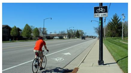
Designated lane for bicycles to travel in the same direction as motor vehicles. Pavement striping, markings and signs are used to identify the bike lane. When riding on a street, a striped bike lane is usually the safest place for a cyclist to ride.
